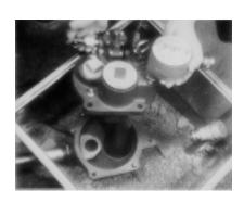
Remove junction box cover and cut 3 electrical splices, disconnect electrical conduit. Lift unit. Replace unit by reversing these steps.
