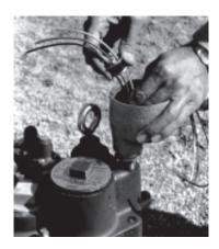
Remove cover from junction box. Feed the 3 motor leads through compression seal. Install compression seal in hole in junction box and tighten two screws.
