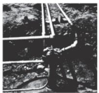
TO TEST PIPING. Block lines at each dispenser. (Trip dispenser shear valve.) Remove line test plug for this test.
