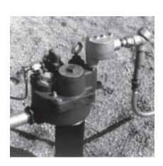
Connect electrical conduit through approved fittings to junction box.
