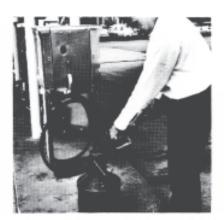
6. After the installation is completed and tests have been made; purge system of air by pumping at least 60 liters through each dispenser. Begin with the dispenser furthest from pump and work toward the pump.
