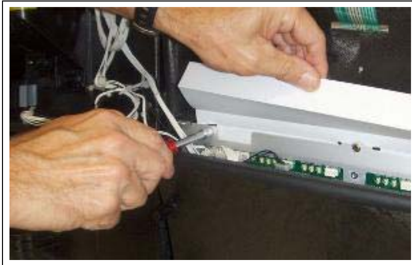
Figure 11: Securing Left Side of PPU Shield
