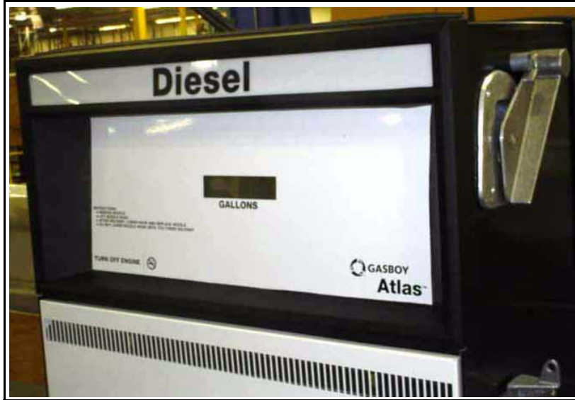
Figure 13: Installation of New Bezels
