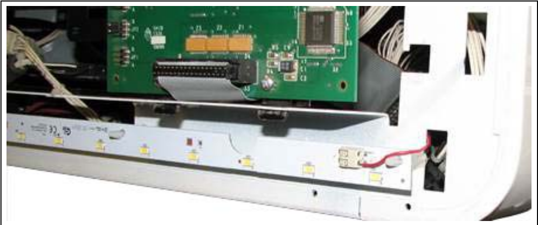
Figure 5: Reconnecting Wires to LED Strip
