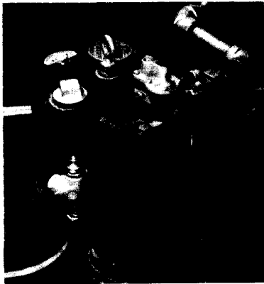
1. Connect electrical conduit through approved fittings to junction box.
