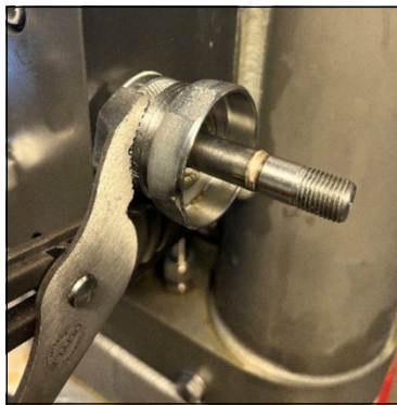
Figure 17. Tightening Outlet Valve to HydrX Manifold
