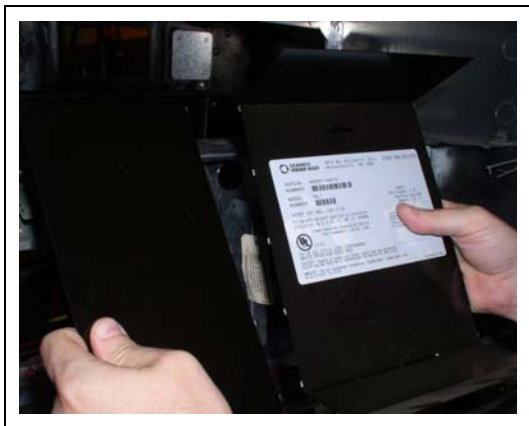
Figure 5: Removing Side Panels of UL Bucket
