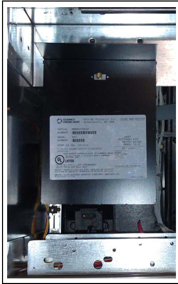
Figure 6: Attaching UL Bucket to T-rail
