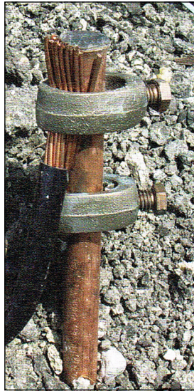
Figure 1. Example - Ground Electrode Installation
