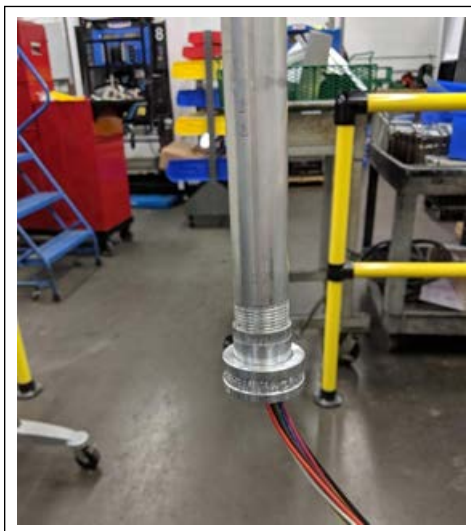
Figure 13: Union on Conduit
