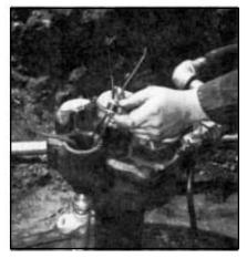
Remove cover from junction box. Provision has been made for 2 wire, or 3 wire and optional ground. Pull wires from power supply through junction box.
