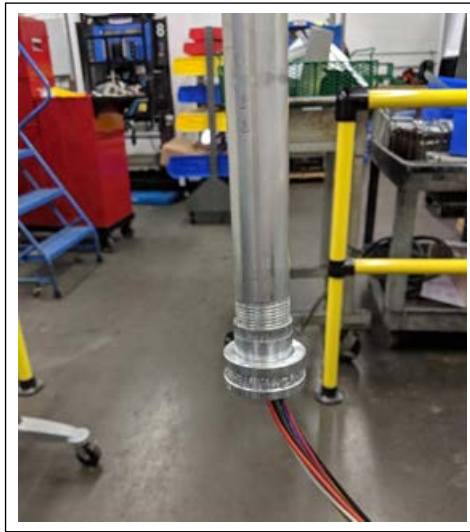
Figure 11: Union on Conduit
