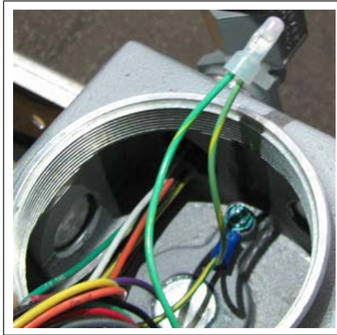
Figure 18: Wire Nut and Ground Wiring
