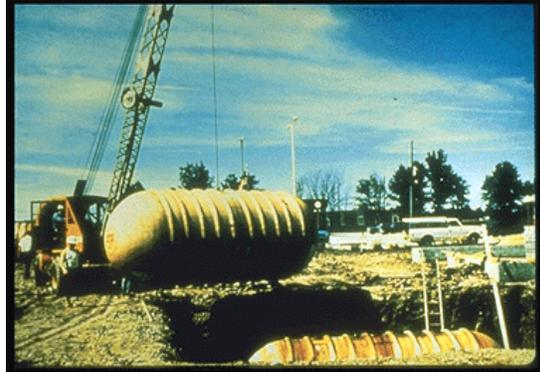
UST components made from metal, however, that routinely contain product and are in direct contact with the ground need corrosion protection provided by cathodic protection or (in some cases) lining the interior of the tank, as described below. These options require O&M.
