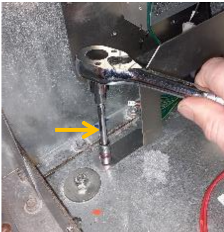
Tighten Mounting Nuts. Vista 4V Wide shown.
