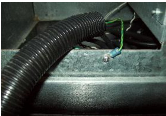
Vista 3V dispenser grounding position.
