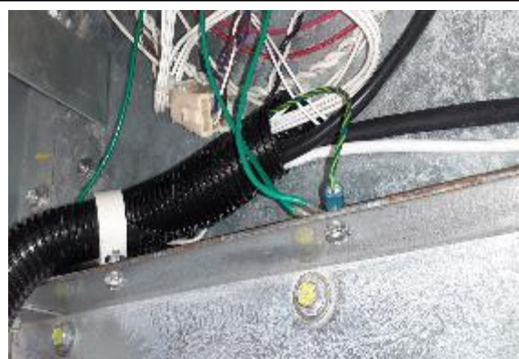
Vista 4V dispenser grounding position.
