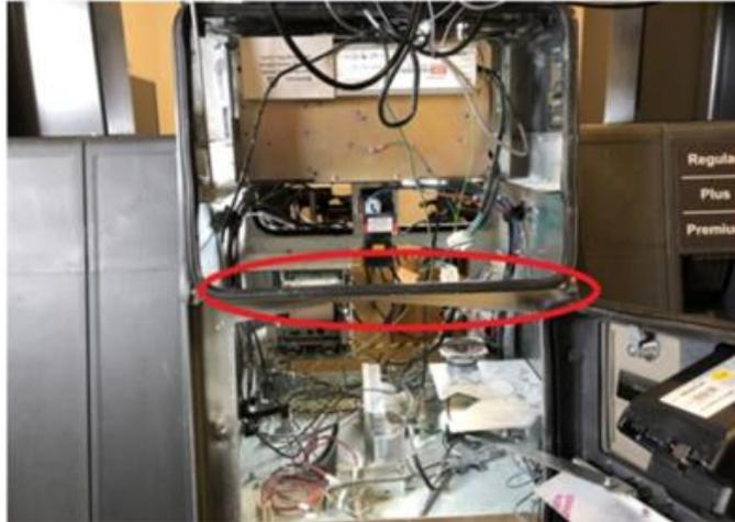
1. Plug in the Low-voltage DC power cable (pre-installed on the PSU assembly), yellow Cat-5e network cable and the Green/Yellow earth cable to the G6-300. If doing a double sided installation, repeat this step for side B of the dispenser.
