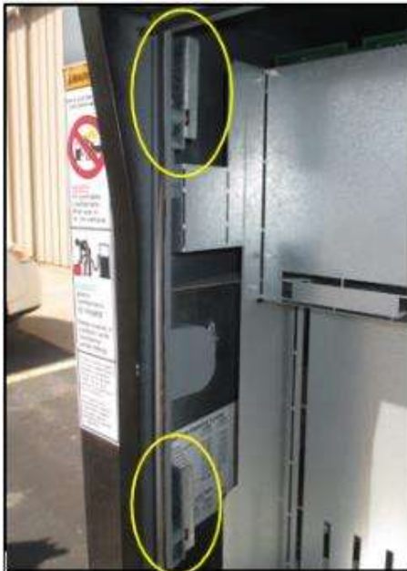
Fig 2.8a – Location of main door latches
