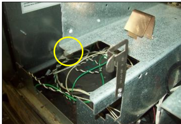
Fig 4.12.2d – Tab snapped off.
