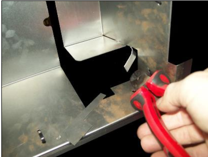
Fig 4.12.3d – Cut off both tabs and discard.
