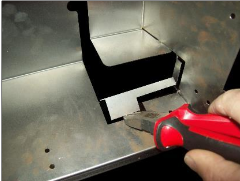
Fig 4.12.4e- Cut off bottom tab and discard.
