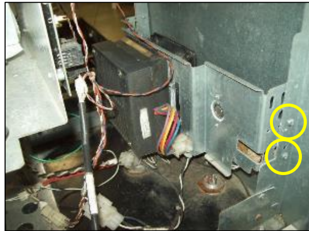
Fig 4.13.1b – Remove Screws Side B.
