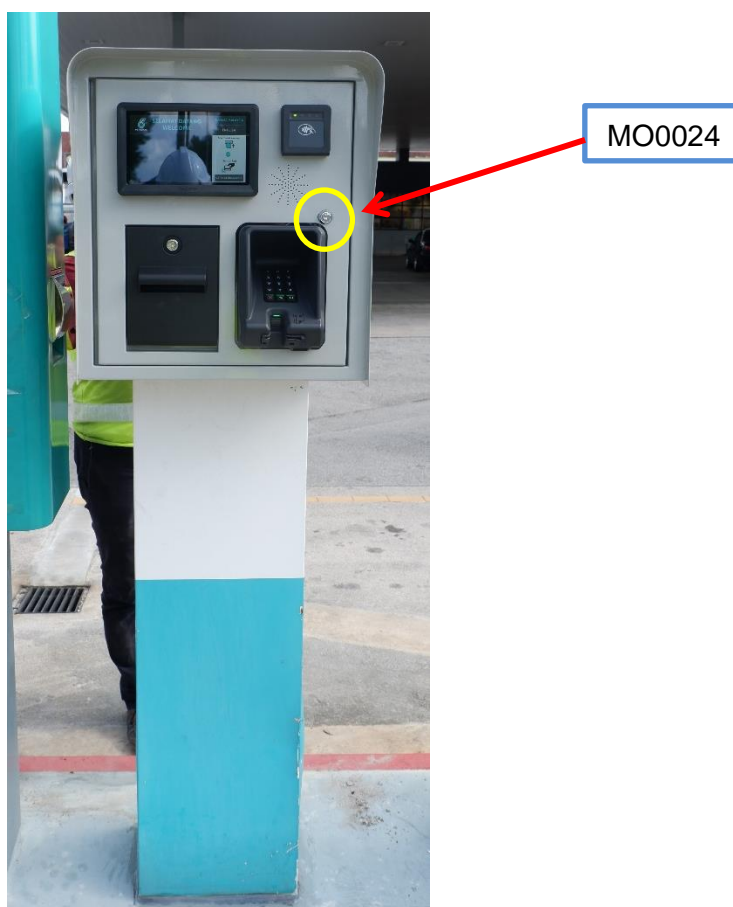
Fig 3.4 – Completed OPT installation for Pedestal.
