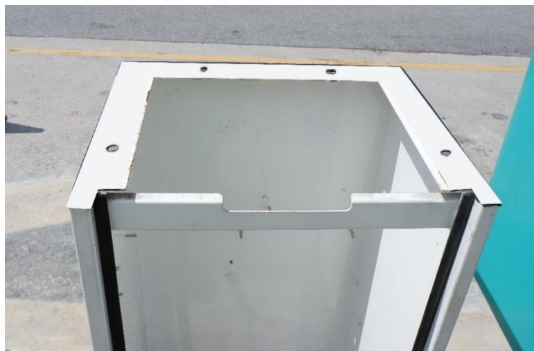
Fig 2.4 – Remove the existing OPT main case and clean the contact surface.
