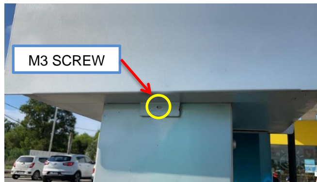
Fig 2.1b – Remove the M3 screw on the highlighted area shows by using a wrench.
