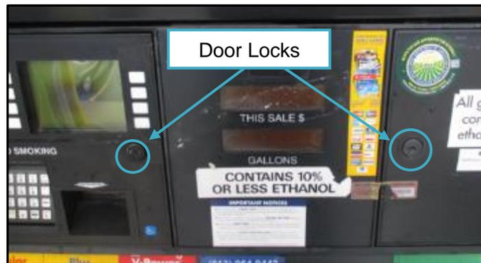
Fig. 1.2a – Unlock both option doors (Wide)
