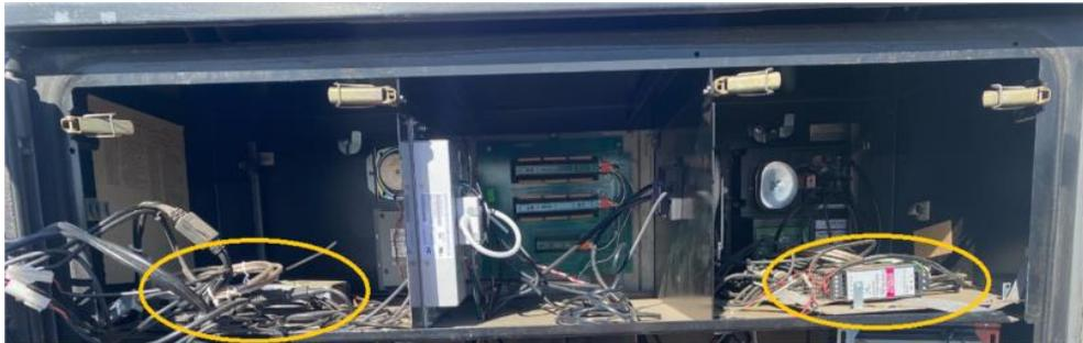
Trace the AC power cable connected to the PSU (circled in below image) to the connection at the other end to identify where this is connected to.
