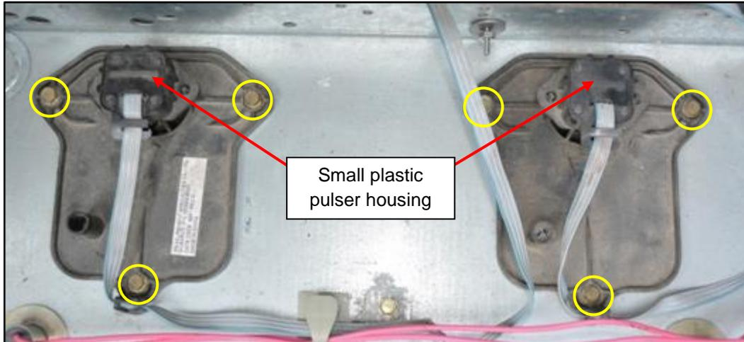
If the pulsers have a small plastic housing on top of a plastic base with 3 screws (circled above), proceed to Step 6.2.2
