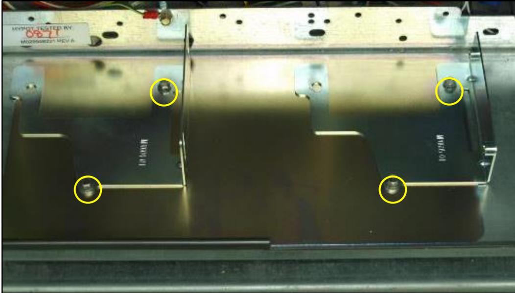
3. Using a 5/16" socket or nut driver, tighten all four MS0166 (or original) screws to secure the Foot Brackets to the cabinet.
