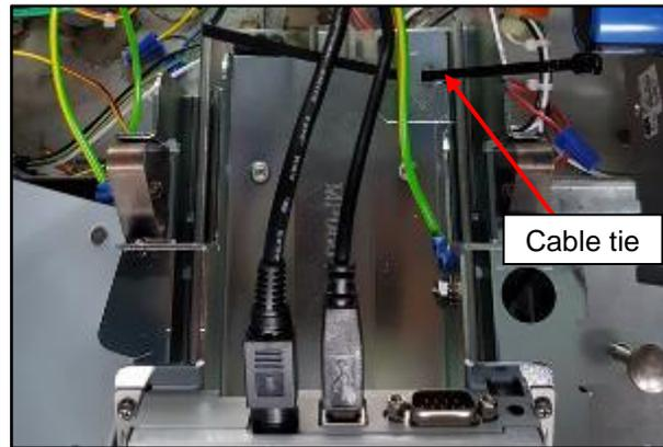
10. Tighten cable tie to hold the cables in the correct location. Cut off the excess cable tie tail.
