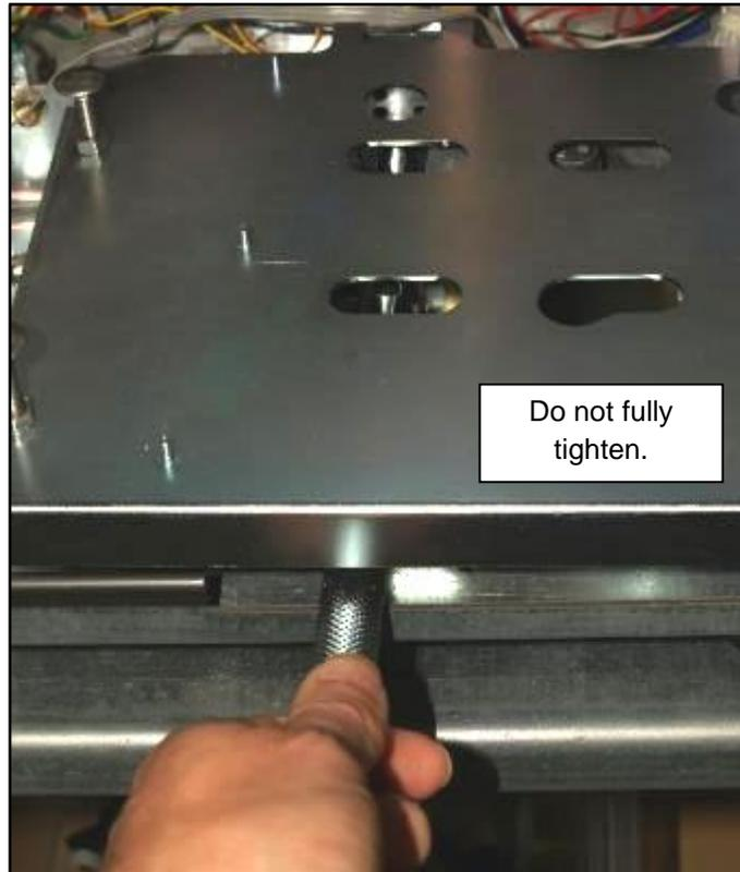
3. Insert two MS0177 M6x12 Sems Screws (circled below) in the right-hand side of the Printer Mounting Platform, threading them into MP0605. Do not tighten the screws.
