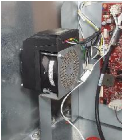
A: Heater (if present). No cables will be disconnected from the heater at this stage.
