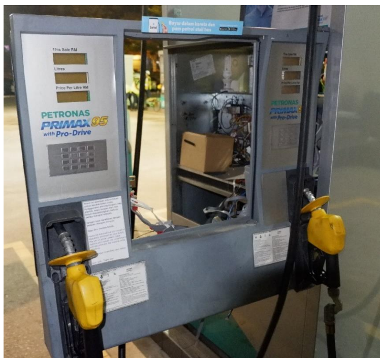
Fig 2.9 e – Remove door from dispenser
