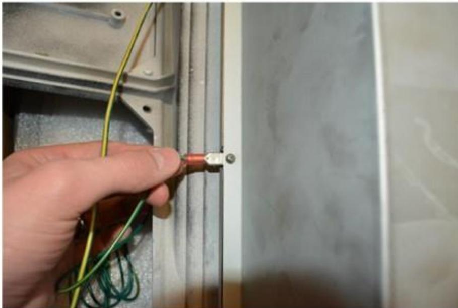
*Attaching grounding cable to shield*
