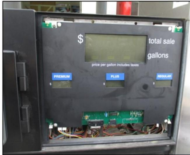
Money/Volume Display assembly re-fastened to Dispenser Frame
